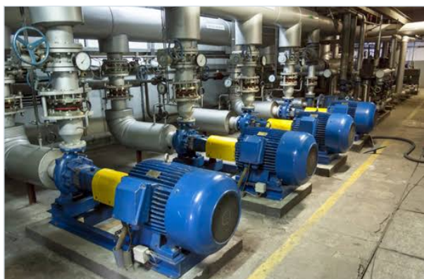
Mechanical plant and pump installation
