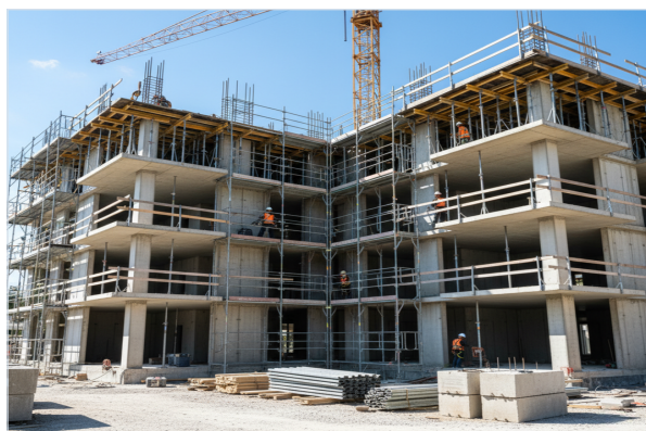
Building and civil construction
